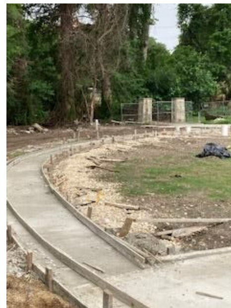
Concrete walk poured around the Dr. Urrutia statue.
