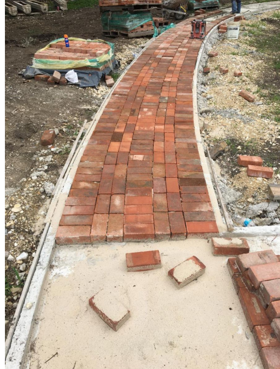
Historic bricks are being re-installed on a sand base by the concrete walk.
